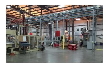
Using existing fixtures and installing Starco LED tubes, all with motion sensors, saved the Berry Plastics Dunkirk plant \$25,000 annually. It improved lighting by at least 30% and qualified for a \$21,000 financial incentive from their electricity provider. A total of 1,157 LED tubes were installed. Starco LED lighting reduced energy consumption by 52%. Occupancy sensors further reduced energy consumption by an additional 25%.
